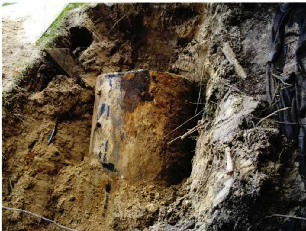
Picture 2: UST 1287Albatross removal in progress.
